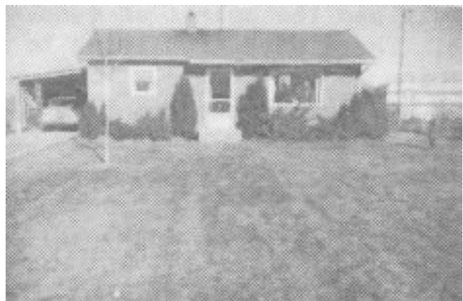
The new house overlooking the river
