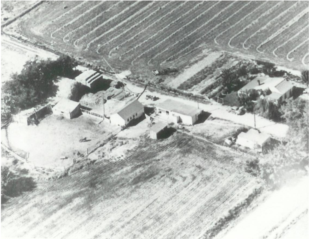
An aerial photograph of the Frost Farm showing the home (left) and outbuildings.
