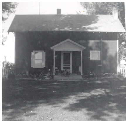
The house on the Story place 550 S 150 E Burley
