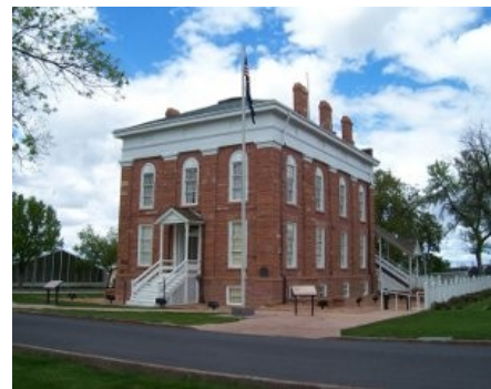
The completed portion. A portrait of Orange Warner hangs in the building
